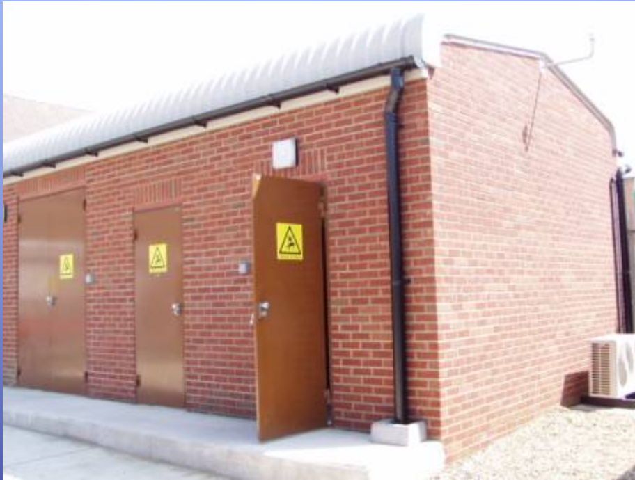
Substation – where the electricity come in.
