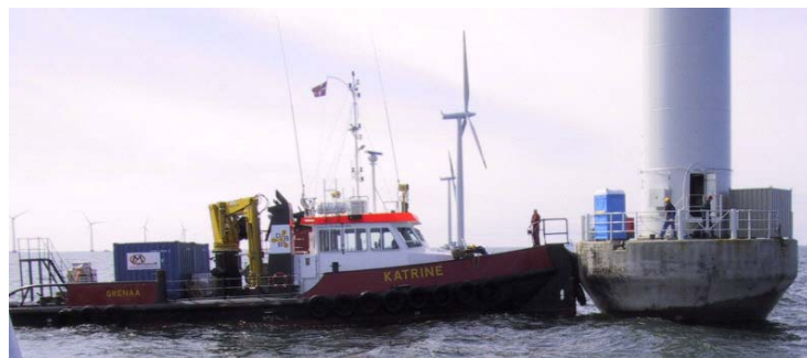
Figure 8-12: Small boat access for operation and maintenance services at Nysted (Source: ENERGI E2 88 ).
