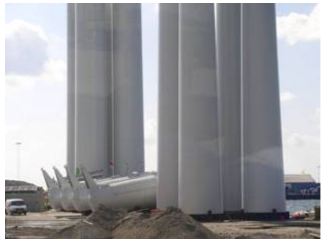
Material at quayside; Source: dena
