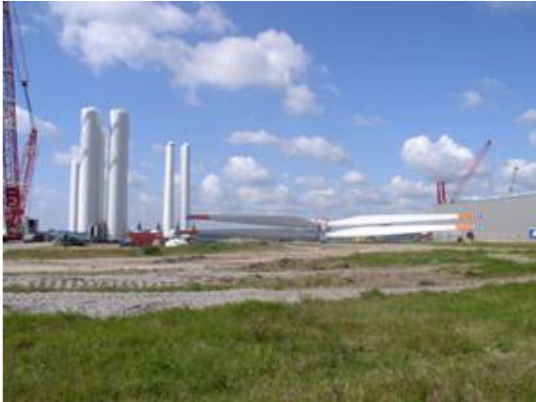
Area for pre assembly; Source: dena
