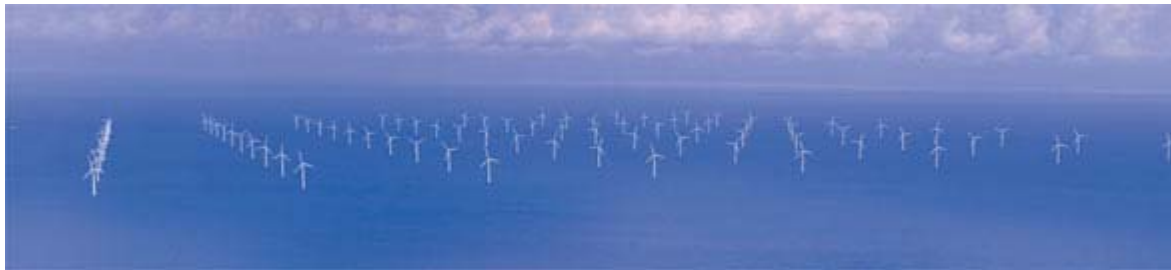
Figure 7-1: View of the Horns Rev wind farm.
