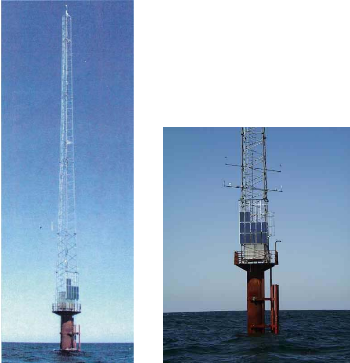
Figure 7-7: Measurement tower at Horns Rev (Source: ELTRA).
