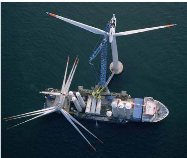
Installation vessel A2Sea; Source: Siemens Wind Power 70
