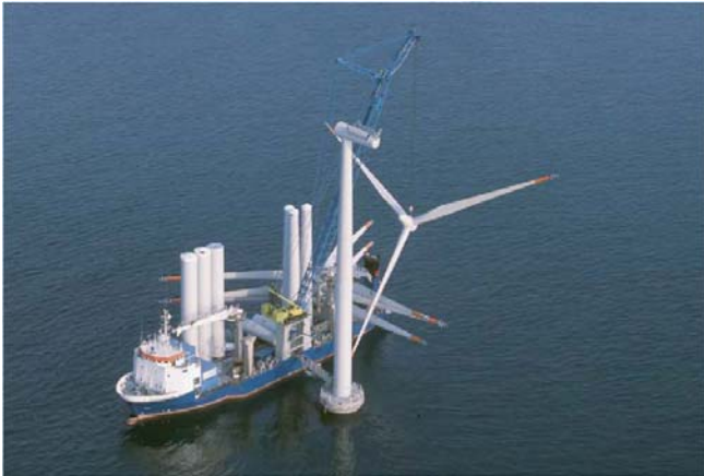
Installation vessel; source: A2Sea Management Report 2003
