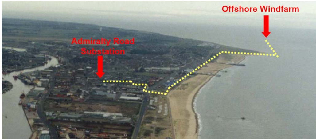
Figure 9-6: Cable to Shore from Scroby Sands Offshore Wind Farm to Substation 121 .
